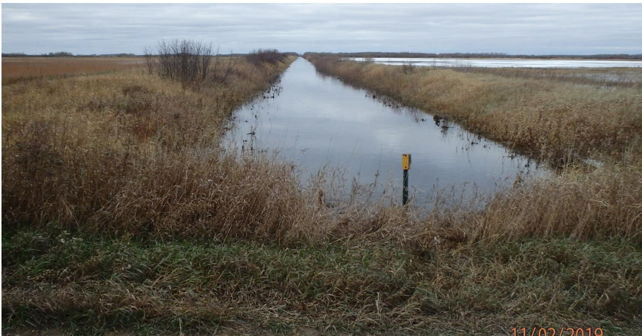
Lat 6 SD 72 – Existing Huseby Pipe looking to the north
