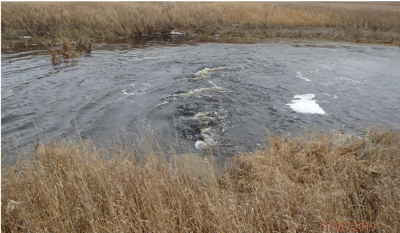
Outlet end of Huseby Pipe into SD 95 Lat 1 Ditch – looking south. Sediment buildup in Lat 1 to be removed.
