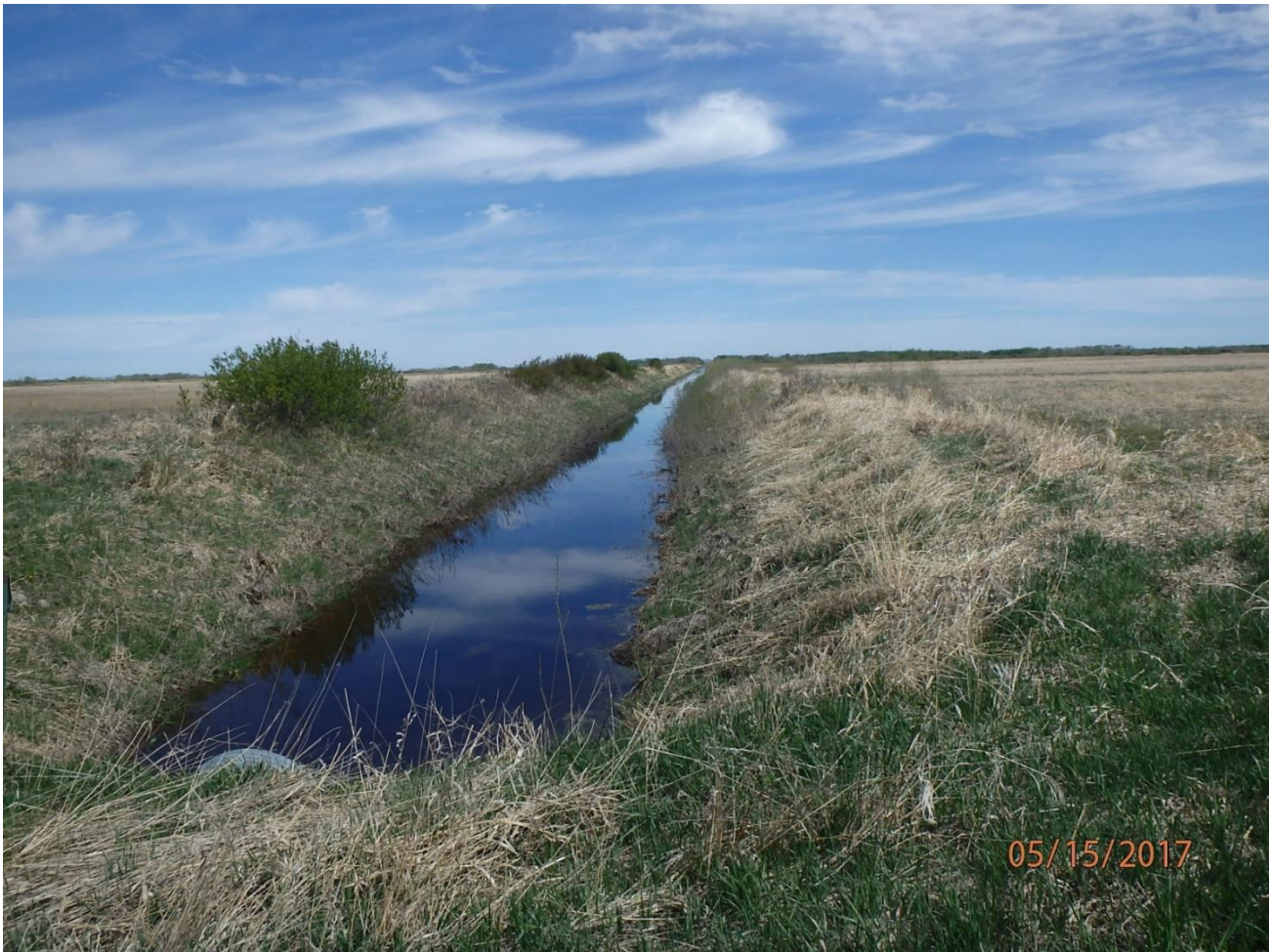
Lat 6 SD 72 – Existing Huseby Pipe looking to the north
